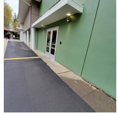
Image 4: River Front Center outdoor space
