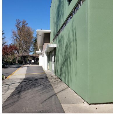
Image 4: River Front Center outdoor space
