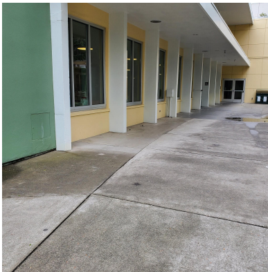
Image 4: River Front Center outdoor space
