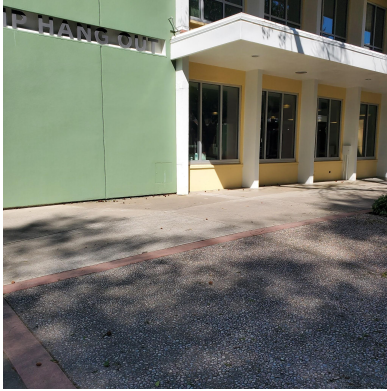
Image 4: River Front Center outdoor space
